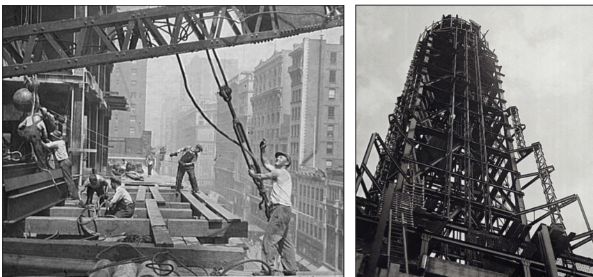
Figura 7. Lewis Hine: construcción del Empire State Building ( http://digitalcollections.nypl.org/collections/ ).
